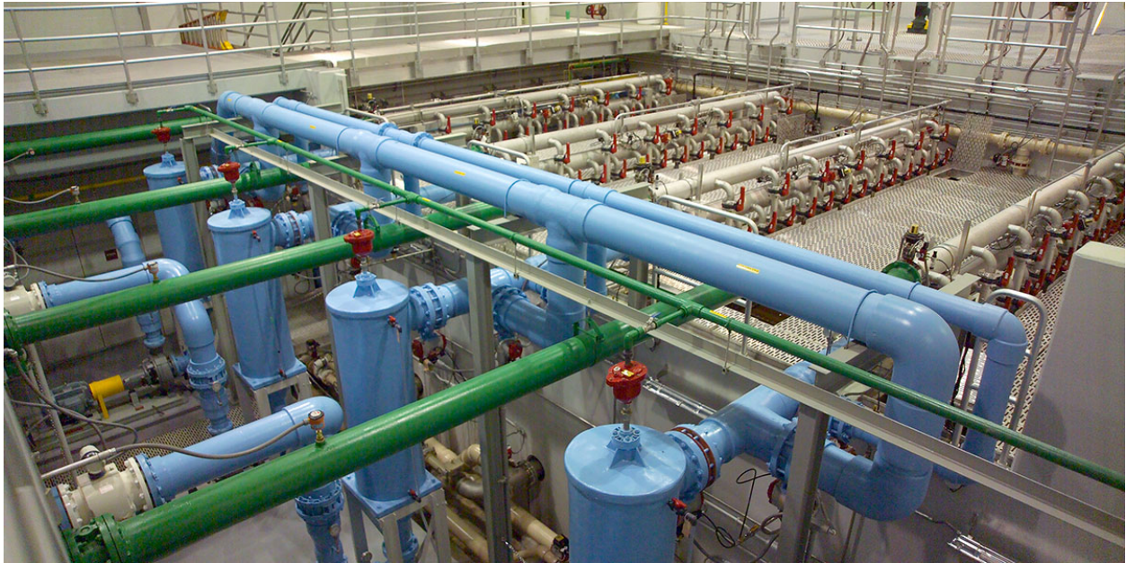
Figure 7: Water and wastewater treatment facility
