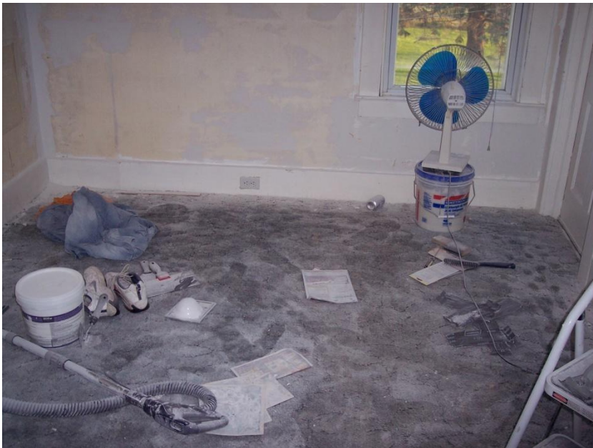
Figure B 4. Sanding of the walls.
