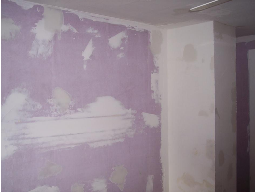
Figure B 3. Resurfacing of the walls.
