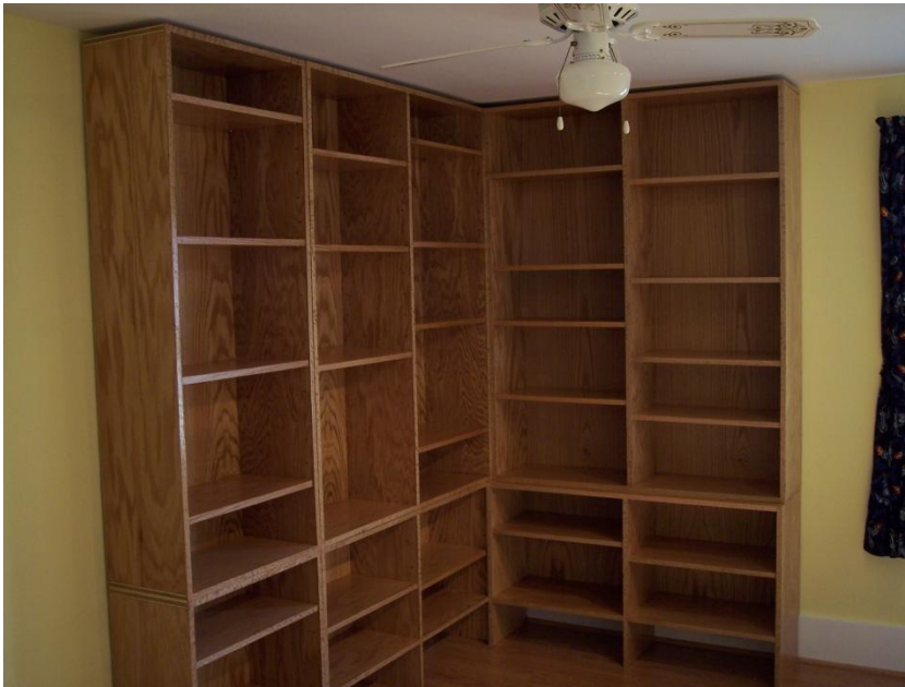
Figure B 9. Dry fitting of nearly completed bookcases.
