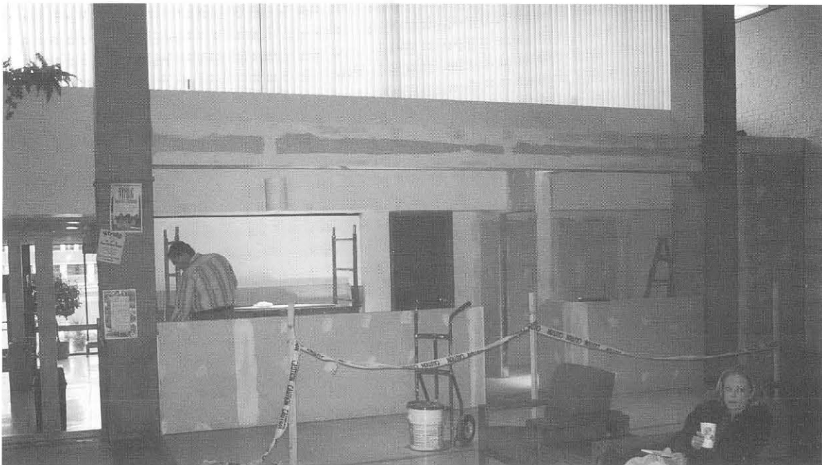
15) Fall '99 students will recall this remodeling job.
