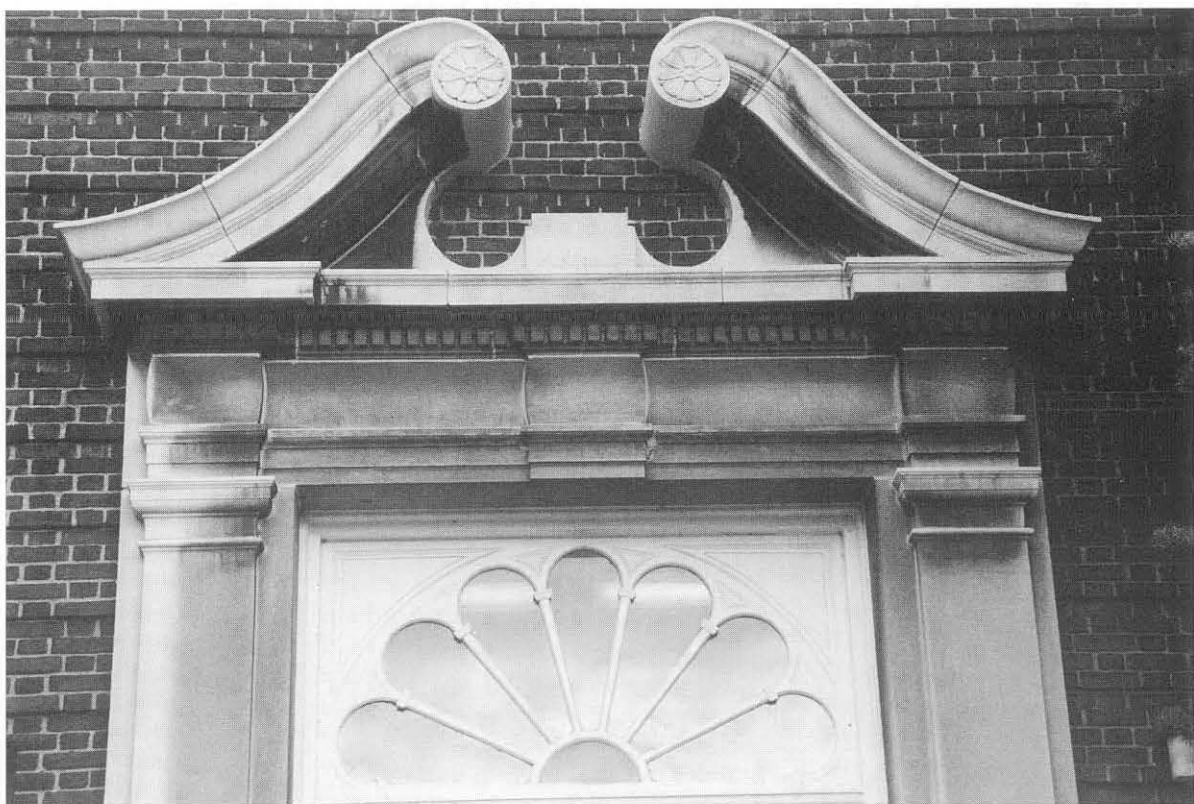
6) This building contains architecture popular in the day it was built.
