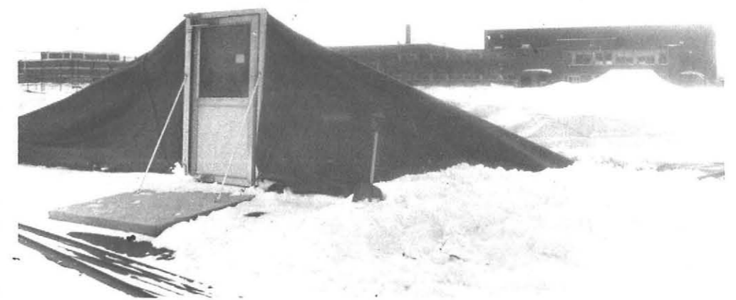
The Bubble Before and after.
