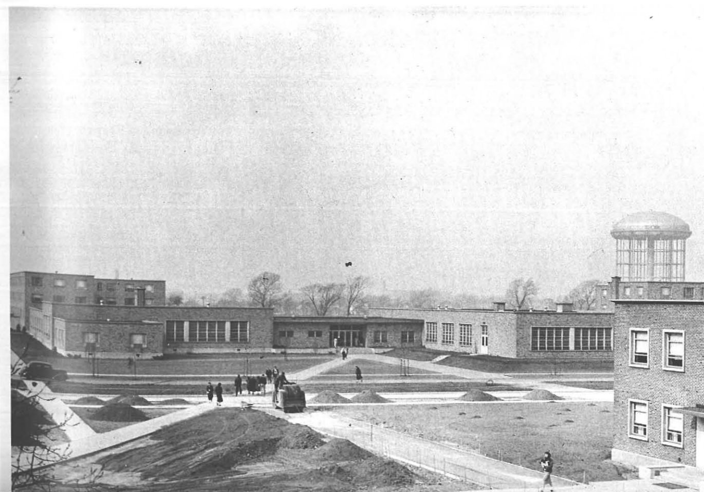
Campus renovation The original Union (center) was the campus' center point in the early 1950's. Construction had just been completed on the original library, far right. The cost of the original Union was $1.5 million.
