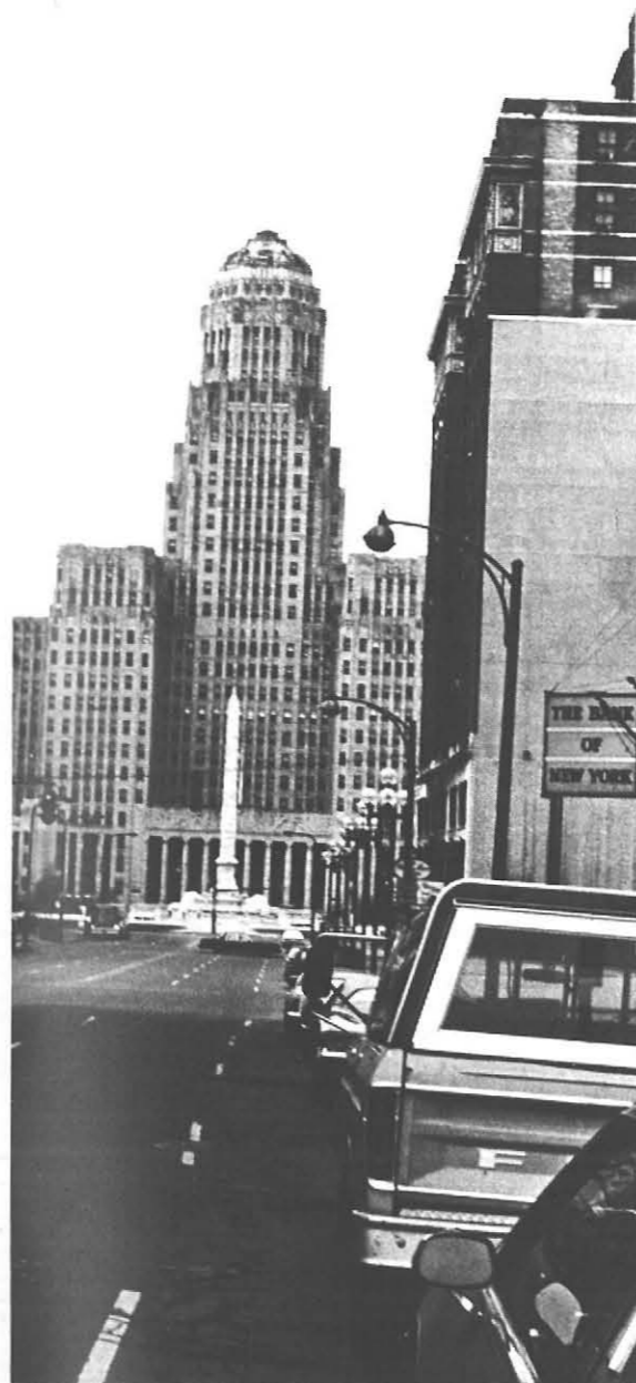
Buffalo City Hall and the McKinley Monument.
