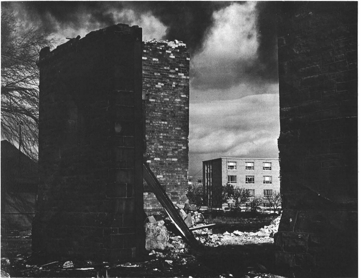
clanking chains, machines that roar . . .
