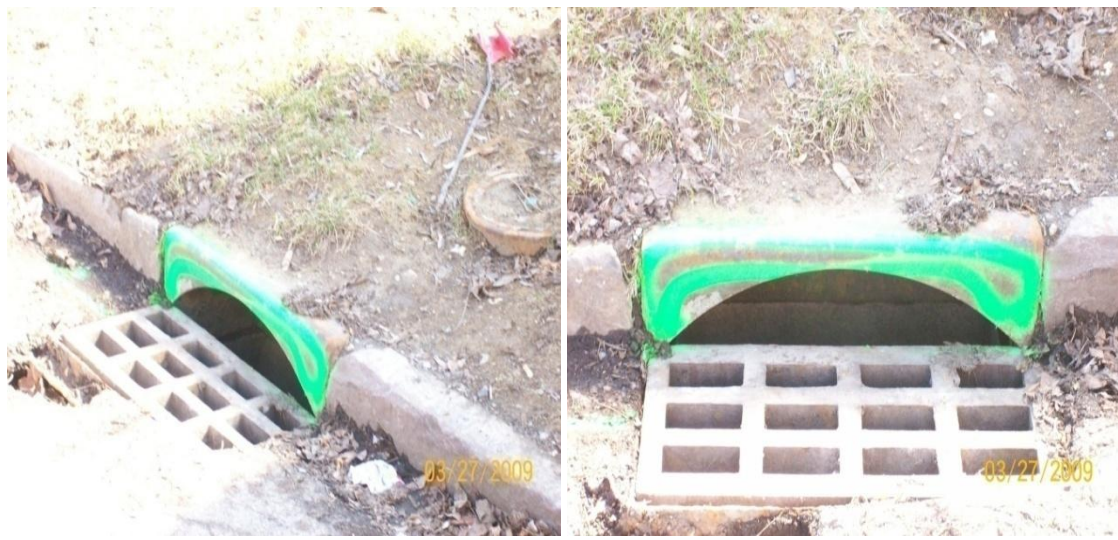
Figure 15. Photo# 15; Figure 16. Photo #16: Spray Painted Sewer Opening
