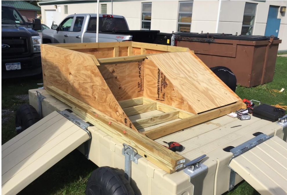
Figure 7. Floating basking/nesting platform in the building process.
