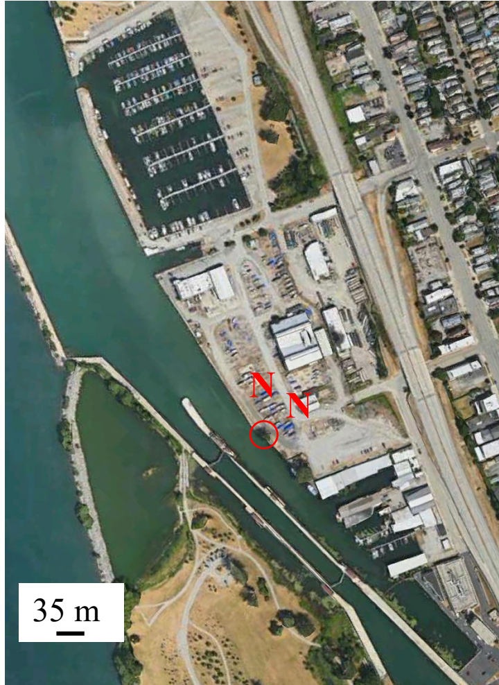
Figure 27. The circle represents the cement ramp that turtles used to access the Rich Marine boatyard. The Ns represent two separate nests found within 50 meters of each other in 2014 and 2016.
