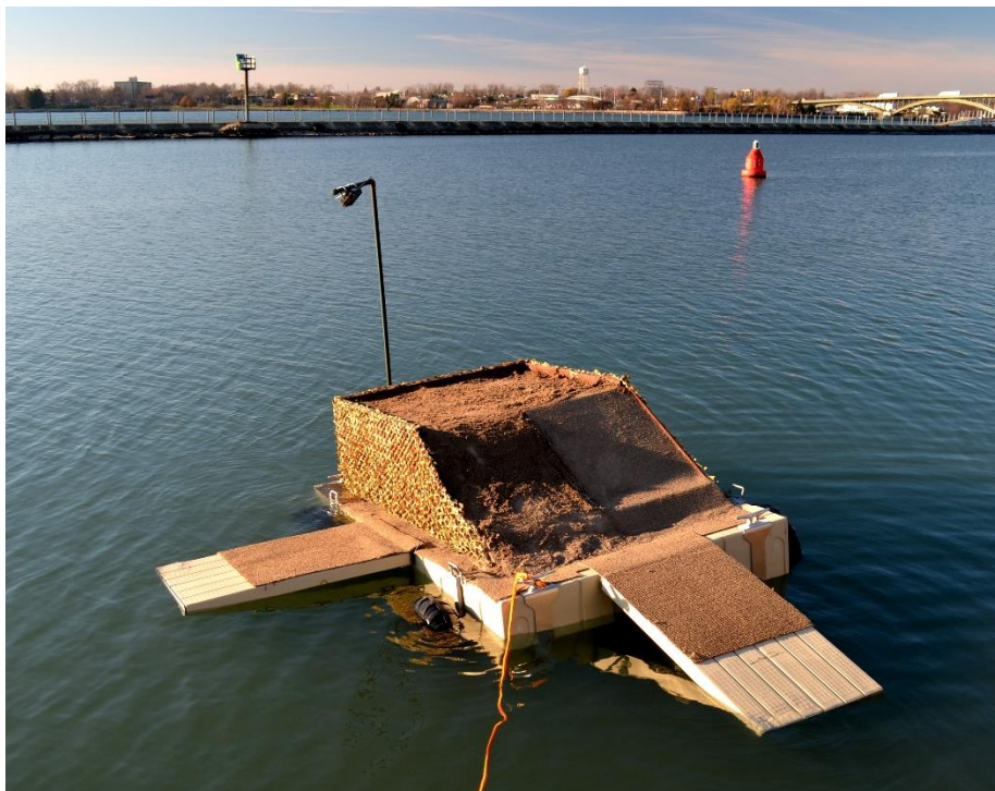
Figure 8. Floating basking/nesting platform design with surveillance camera mounted above.
