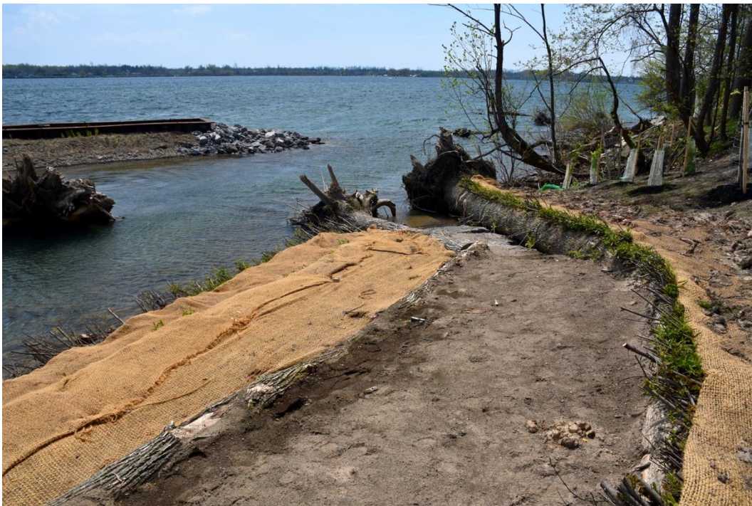
Figure 31. Riparian restoration on Little Beaver Island that incorporated characteristics of turtle nesting habitat.
