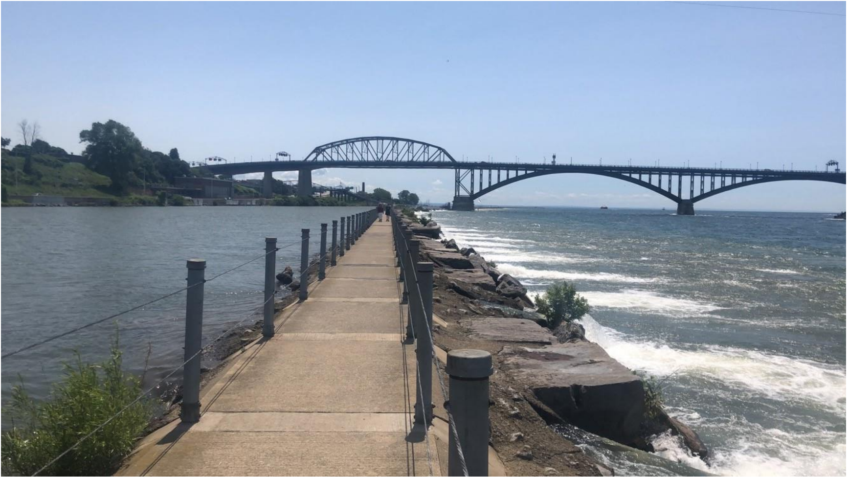
Figure 30. Culverts that allow flow between the Black Rock Canal and the upper Niagara River.
