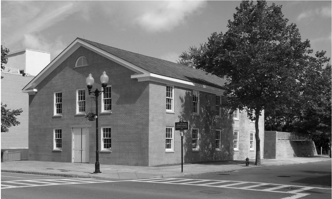
Figure 3. Wesleyan Chapel, site of first Women's Rights Convention, Seneca Falls, N.Y. 1848, www.nps.gov
