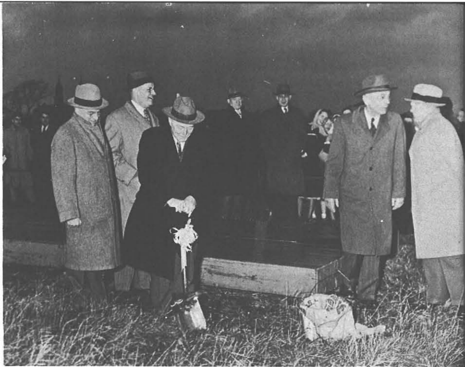
Breaking the ground, designating the culmination of years of effort and planning.
