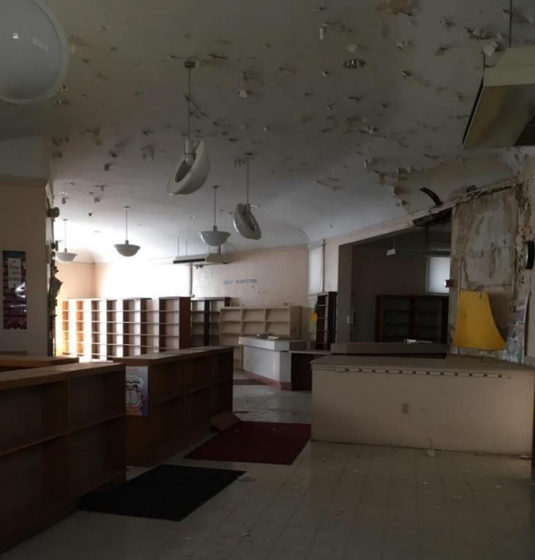
Fig. 6 Inside 2351 Delaware Avenue
