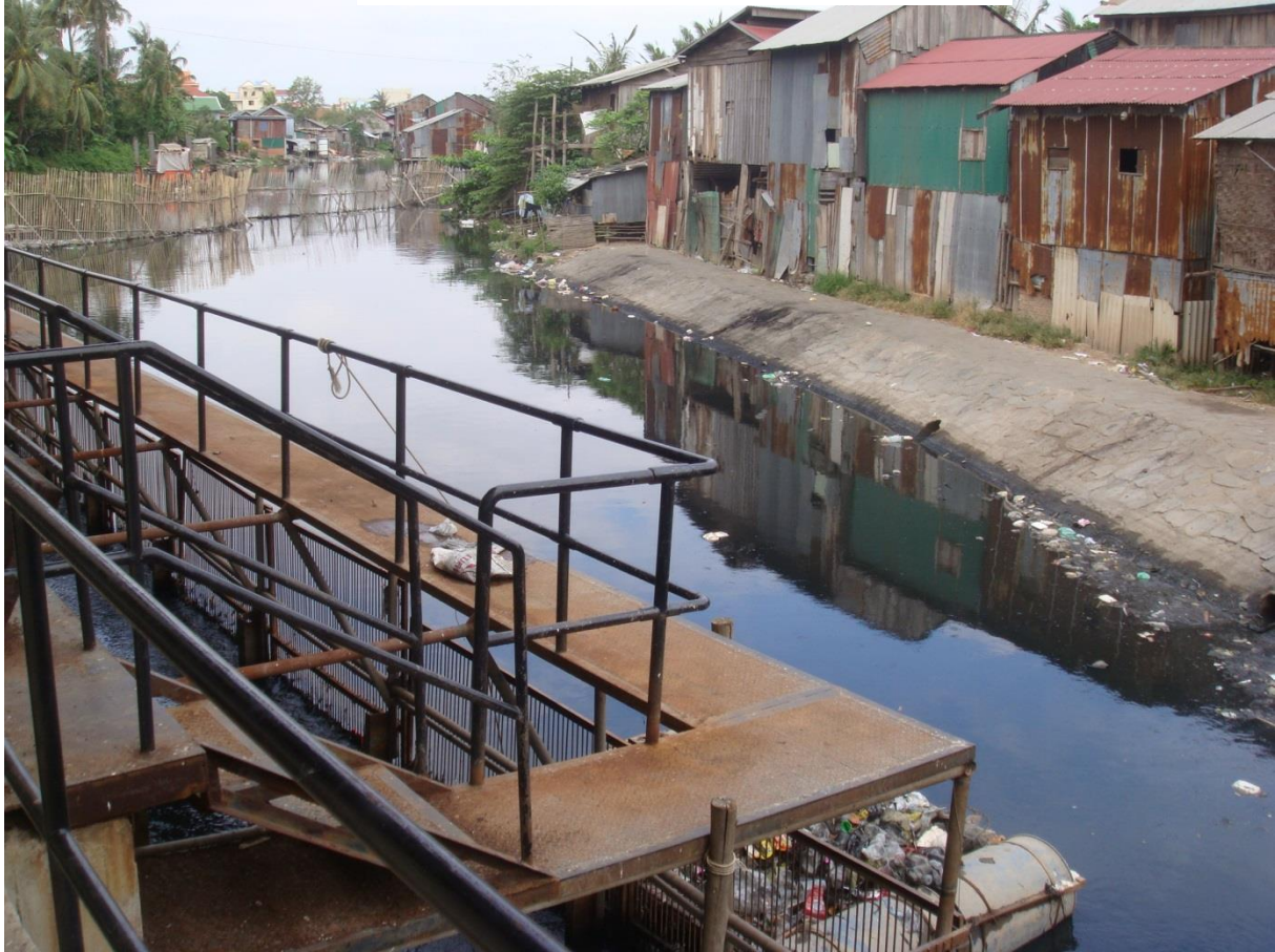
Figure 11. Squatter housing behind the Tum Pun pump station (T2P).
