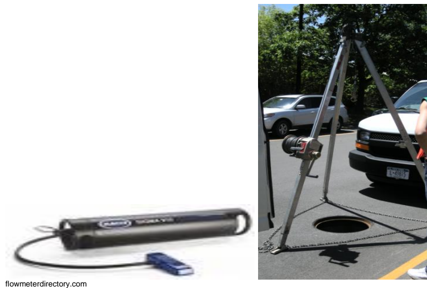
Figure 3.4: Sigma 910 Flow Meter Installation. A 7.8 lbs, 4.5in x 17.625in Sigma 910 flow meter was installed inside manhole #230 on Rockwell Road using a harness apparatus to lower maintenance crew inside the manhole.
