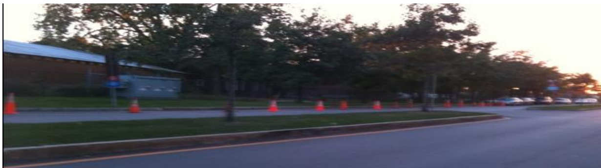
Figure 3.2: Rockwell Road upstream and downstream (left side) of Stormceptor. This is a two lane road in both directions. One lane is blocked off so sampling can be performed since both the upstream and downstream sites are located on the road.
