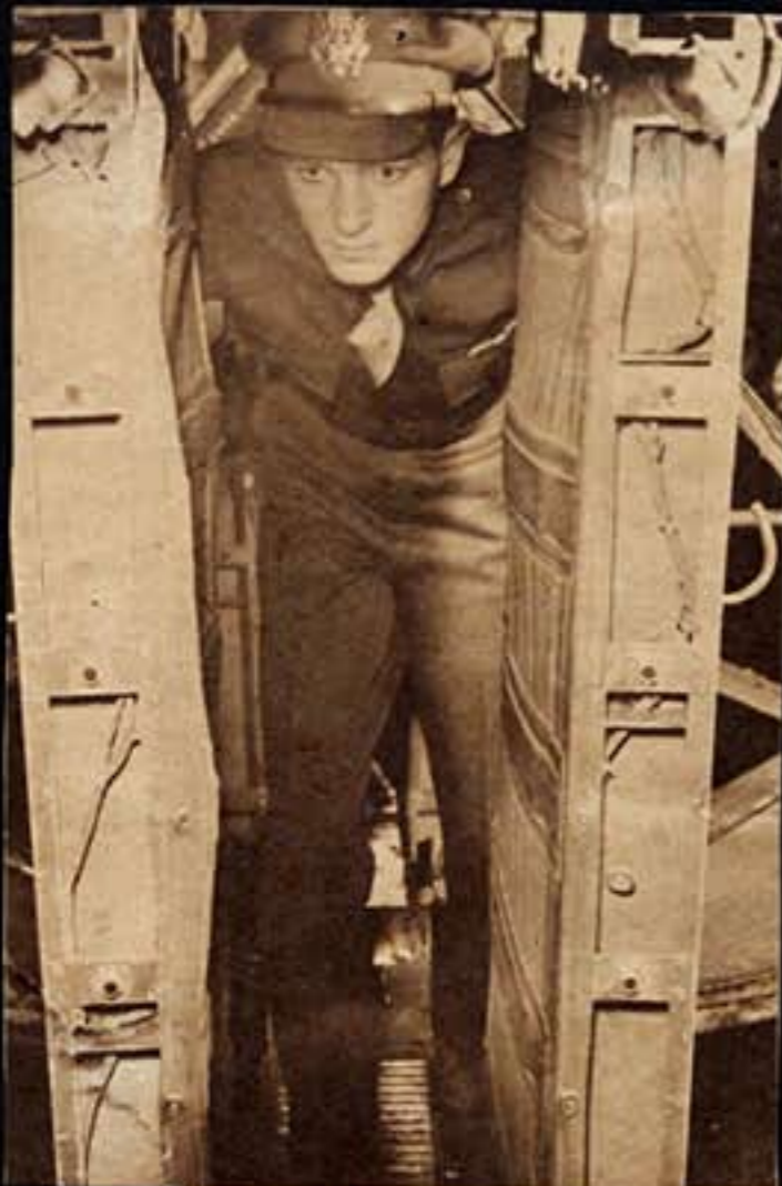
THE B-24 IS BIG, but there's so much aboard that it's a tight squeeze in a lot of places. The pilot enters through the bomb bay doors in the ship's belly, climbs to a catwalk between the bomb racks, and from there pulls himself up to the flight deck, where his controls are located. Climbing aboard is Lieut. Wilfred E. Moran of 70 Norman Ave., a former student at South Park High School and State Teachers College.
