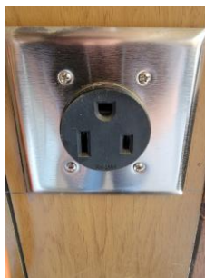
Figure 11: NEMA 6-50 Outlet. (Own photo, 2021)
