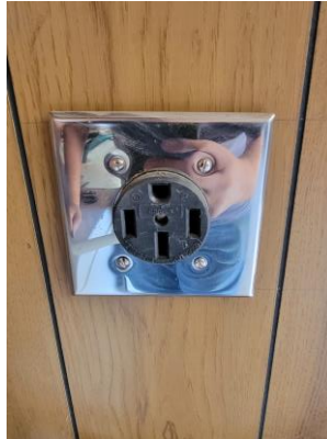
Figure 10: NEMA 14-50 Outlet. (Own photo, 2021)
