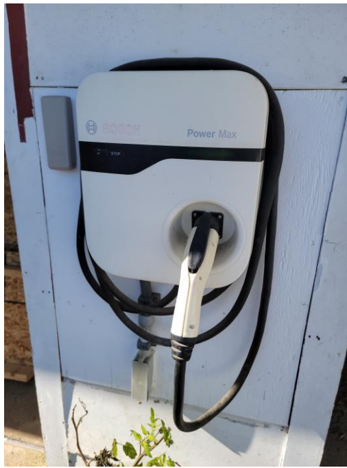
Figure 2: J1772 Plug, Level two charger, Bosch Power Max Charger – Home Install. (Own photo, 2021)
