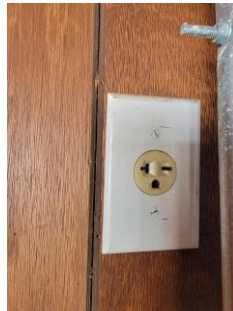
Figure 13: NEMA 6-20 Outlet. (Own photo, 2021)
