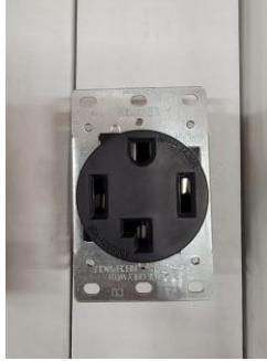
Figure 12: NEMA 14-30 Outlet. (Own photo, 2021)
