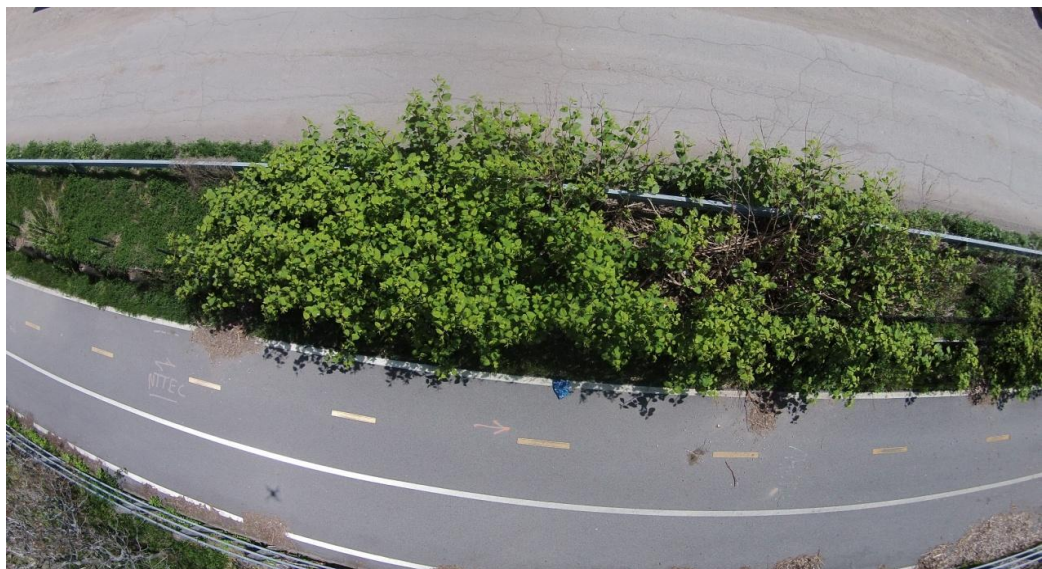
Figure 13 The original image of the site near the Peace Bridge.
